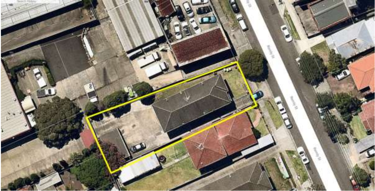
Figure 11: Aerial of 1 Remly Street
